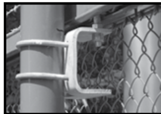
ISTB - Internal Slide Gate Track Bracket
